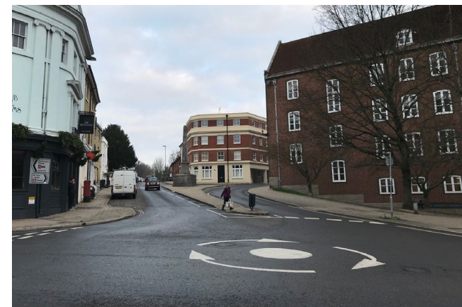
Figure 3.11: Junction of Romsey Road at Westgate
